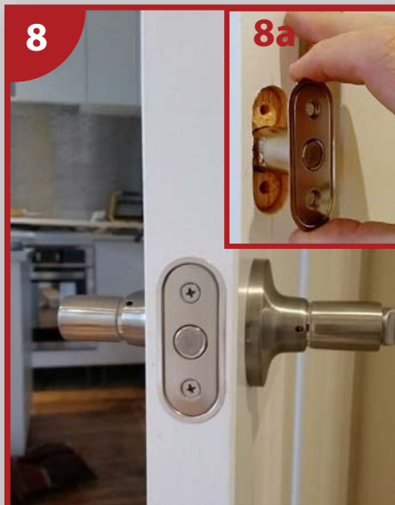
8. Insert latch assembly into the door edgebore hole (8a) and secure in place with screws provided. Be careful not to over tighten screws as this may cause the flanged housing cups to deform and/or cracking in timber. Note: screwheads must fit below, or perfectly flush to the surface of the latch/strikeplate, to allow coverplates to adhere properly to surface (FIG. A). Now install chosen door handles as per manufacturers instructions.
