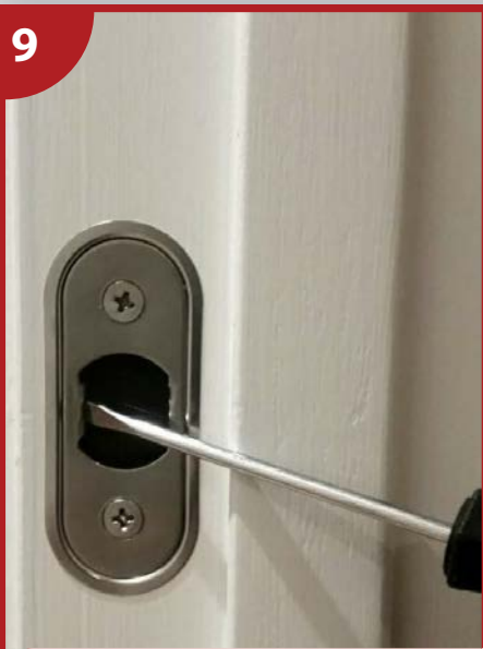
9. Insert the strikeplate assembly (incl. strikebox/drilling template) into the prepared jamb 'cutout' so that the latch/bolt rests against Adjustment Tab A when in the locked/latched position (FIG. C). Secure in place with screws provided. Test door operation and if necessary 'bend out' adjustment tab with the AM60 ITP screwdriver (FIG. B), to reduce latch/bolt rattle.
